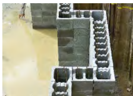
STEPOC in a basement level application
