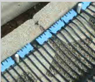
Keystone block showing grid connection
