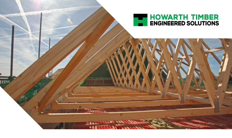
The Howarth Timber Engineered Solutions design and production process is fully integrated. This generates the necessary geometric profiles, the appropriate timber grade and section, and type and size of connector plate. A semi-automated manufacturing process establishes the truss profile by positioning within a range of jigs and press types, which are selected to reflect the complexity and size of the truss. Where required, timber can also be preservative treated.
