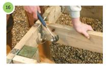
After treating the cut ends of the joist with End-grain, nail in place into the joist hanger. If you are using the contemporary handrail system you can now start to fix your deck boards.
