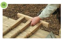
Lay the spindles flat and attach the bottom rail using the galvanised or stainless steel screws.
