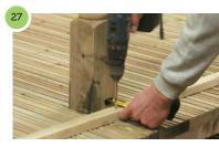
Once all the boards are fixed, determine the position of the edge of the deck. Attach a baton as a temporary guide line.
