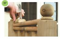
Gently knock the finished rail into place. Use an offcut to prevent damage to the rail.
