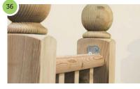
To prevent the top bracket being seen, fix the bracket so the vertical plate is above the top rail.
