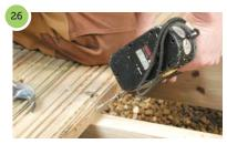
Skew screw through the side of the deck board to attach the board to each joist. If necessary pre-drill at the ends of the boards to prevent splitting.
