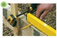
Adjust the height of the side beams to allow a slight fall in the deck away from the house. This will ensure the deck drains correctly.
