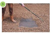
Cover the area with 50mm depth of gravel. Determine the position of the support posts. Dig a hole 600mm deep and 600mm in diameter. Fill with concrete and leave to set for at least 24 hours.
