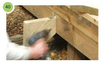
Secure the stringer by skew screwing to the beam or using a framing anchor.
