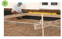
Using temporary braces for support attach the beams to the ledger. Allow for some adjustment to ensure the deck will be square and level.
