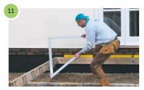
Check the beams are square using a 3, 4, 5 square, reinforcing all the corners using a framing anchor.
