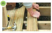
Push each board against the previously fixed board. The deck clips should fit under the fixed board. Whether using deck clips or screws you should always employ a minimum gap between boards of 6mm.
