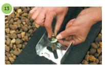
Accurately position the post bases and attach using expanding bolts.
