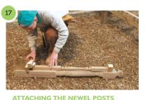
Calculate the height of the handrail by placing all the components on the newel post. Mark the height of the top of the joist.
