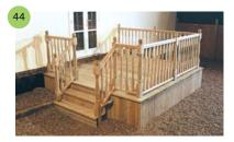
The finished deck fitted with the Arbordeck classic handrail. The sides of our deck have been cloaked with deck boards. Adequate ventilation has been provided to allow the substructure to dry after rain.
