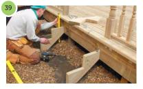
Checking for the vertical attach the furthest stair stringer.
