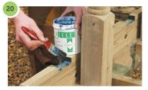
LAYING THE DECK BOARDS After carefully marking the boards notch out positions for the posts and treat with Endgrain.
