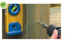
Holding the post vertical and with your mark at deck level, attach the post using the landscape screws.
