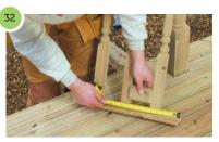
Use a spacer to ensure that the spindles are evenly spread. The maximum gap between the spindles must be no more than 100mm.
