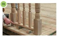
Use supports to help ensure the rail is level. Make sure there is sufficient space to fit the bottom angle brackets. Ensure the gap between the deck board and base rail is no greater than 100mm.
