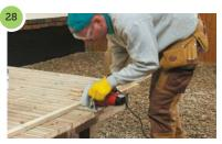
Using the guide line trim the excess board with a circular saw. Remove the guide baton.
