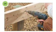
Attach the posts to the beams using coach bolts or landscape screws.
