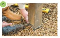
Where possible make sure the original treated end of the post is on the ground and attach using galvanised or stainless steel screws.
