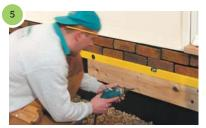
After cutting to length attach the ledger to the wall with suitable bolts. A 10mm gap should be spaced between the wall and the ledger to ensure drainage.
