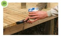
Don't forget to brush the cut ends with Endgrain preservative.
