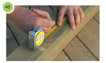
The top of the handrail should be 900mm from deck level. Mark this height on the newel post.
