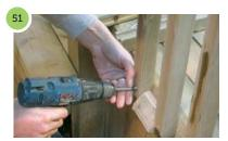
Calculate the spacing required on each spindle (max 100mm) and attach using a spacer as a guide.
