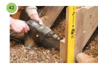
Holding the newel post vertical attach using landscape screws. Remember this post is resting on the ground and so should be supported by a concrete pad and post base.
