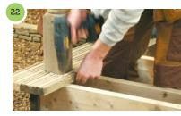
Attach the first two boards by screwing through the surface using galvanised or stainless steel deck screws.
