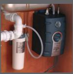
The hot water boiler and initial filter are included with the tap.
