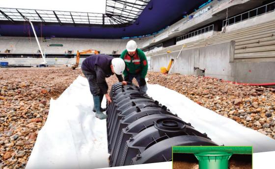
An attenuation system works when the peak inflow rate in a storm exceeds the allowed discharge into the watercourse. The excess flow has to be 'attenuated' by storing the water on the site for the duration of the storm. This is then released at, or less than, the allowed discharge rate after the storm.
