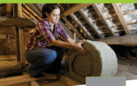
Sheep's wool insulation can be used as an alternative to conventional insulation in walls, floor and roof.
